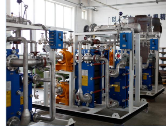
Water /Glycol unit
