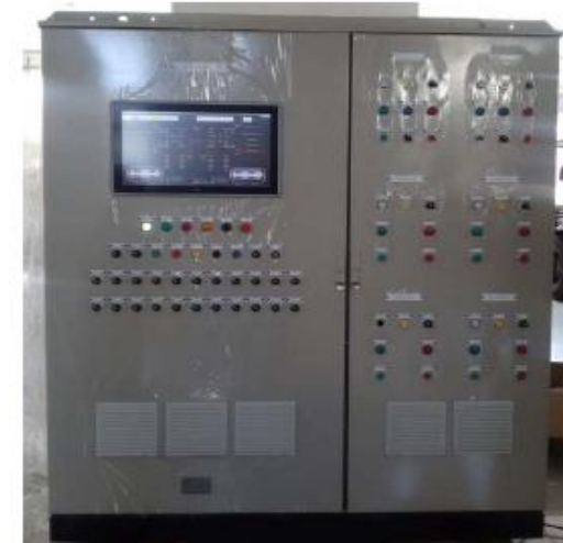
FGSS main control cabinet
