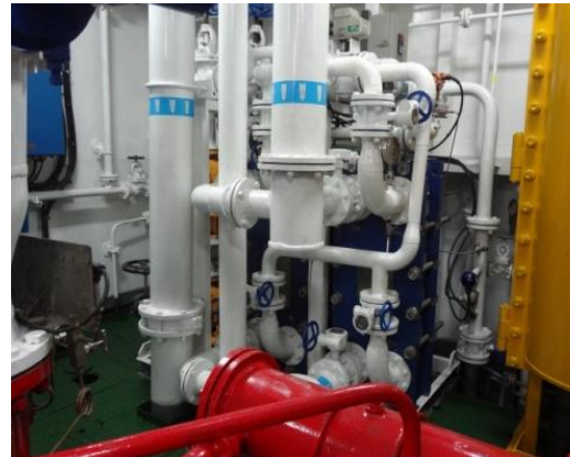
Water /Glycol unit
