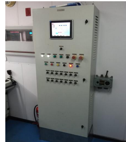
FGSS main control cabinet
