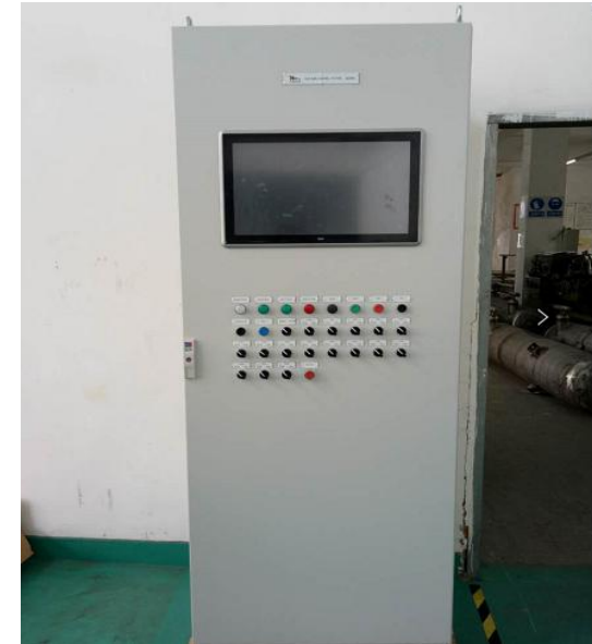
FGSS main control cabinet
